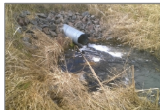
Figure 1. Upstream Drainage Tile Outletting into Restored Wetland
