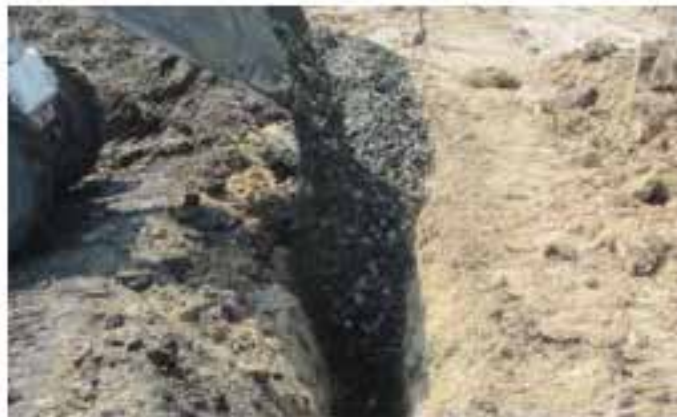
Figure 4.5.31 Construction of Aggregate Barrier
